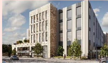
Mandela Way, Southwark Planning status: Submitted Size: 144,000 sq ft Earliest start on site: Q4 2023 GDV: £92m
