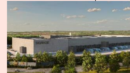
Thurrock Planning status: Submitted Size: 644,000 sq ft Earliest start on site: Q1 2025 GDV: £225m
