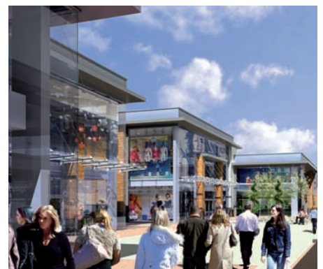
↑ The 302,000 sq ft retail development at Whiteley Village in Fareham is designed to be 35% more carbon efficient than current standards and to achieve BREEAM Excellent. We intend to incorporate 2,850 sq ft of photovoltaic panels and will provide occupiers with Green Building Guides.
