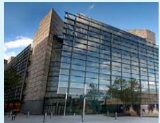
1 Triton Square 369,000 sq ft Completed Q2 2021
