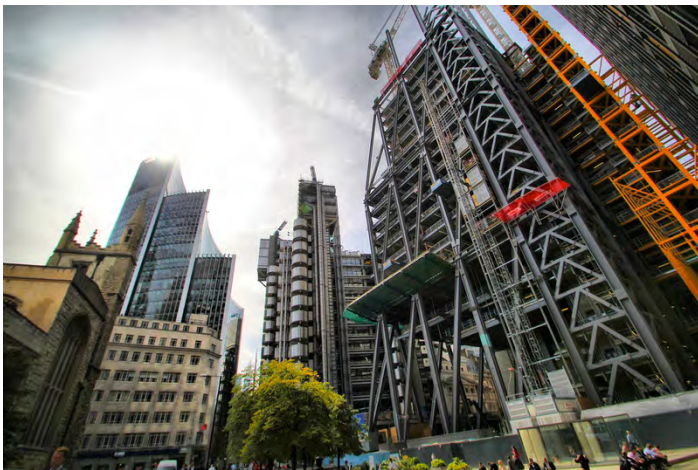
Construction underway at The Leadenhall Building in September 2012.
