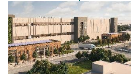
Heritage House, Enfield Planning status: Consented Size: 437,000 sq ft Earliest start on site: Q4 2025
