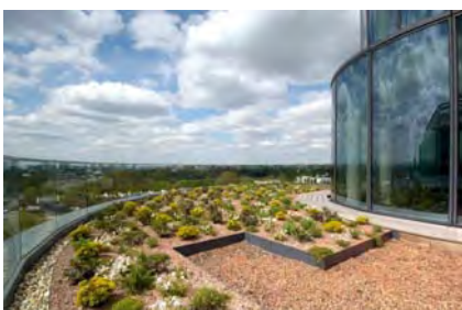
The green roofs at 10 and 20 Triton Street
