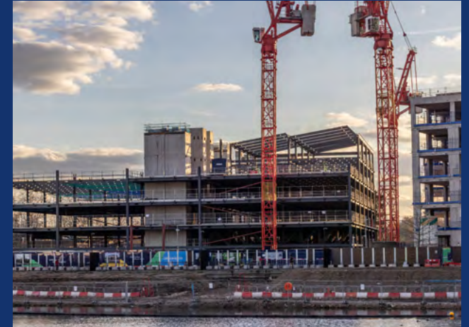
Canada Water, The Dock Shed A2
